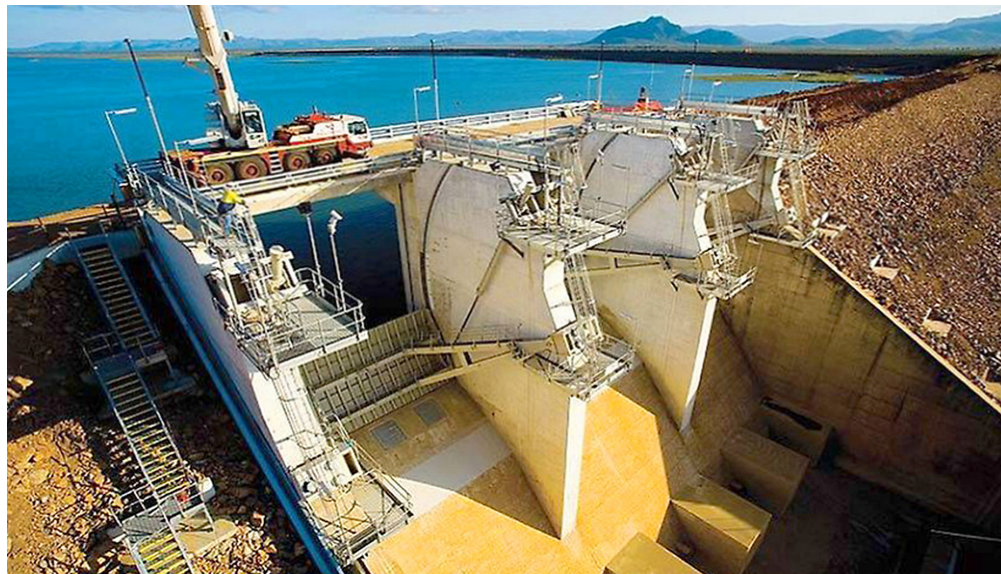
Spillway gates on the Ross River Dam following the 2007 upgrade.
