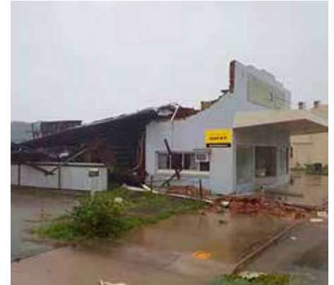
A badly-damaged plumbing business in Proserpine, 101km north west of Mackay.
