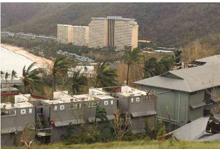
Hamilton Island roof damage.
